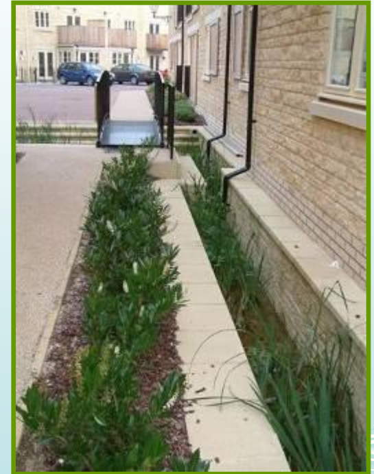
SuDS scheme at Stamford Robert Bray Associates
