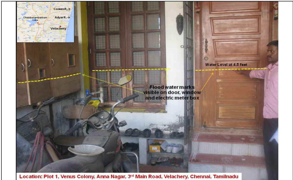
Fig-17 Flood water mark observed in doors, windows and electric metre box due to discolouration in one of the houses at Plot 1, Venus Colony, Anna Nagar, 3rd Main Road, Velachery. (c) NRSC/ISRO, 2015
