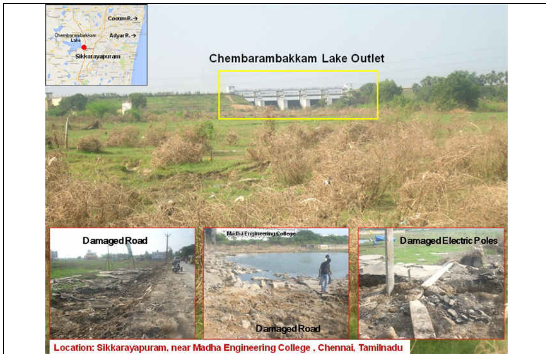
Fig-11: Flood damage to road and electric poles suffered due to gushing flood water at Sikkarayapuram (Kancheepuram district), near Madha Engineering College. (c) NRSC/ISRO, 2015
