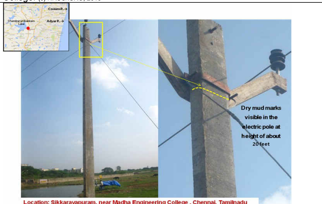
Fig-12 Layers of dried mud marks clinging to electric pole indicating height water attained on December 2, 2015 at Sikkarayapuram (Kancheepuram district) near, near Madha Engineering College. (c) NRSC/ISRO, 2015
